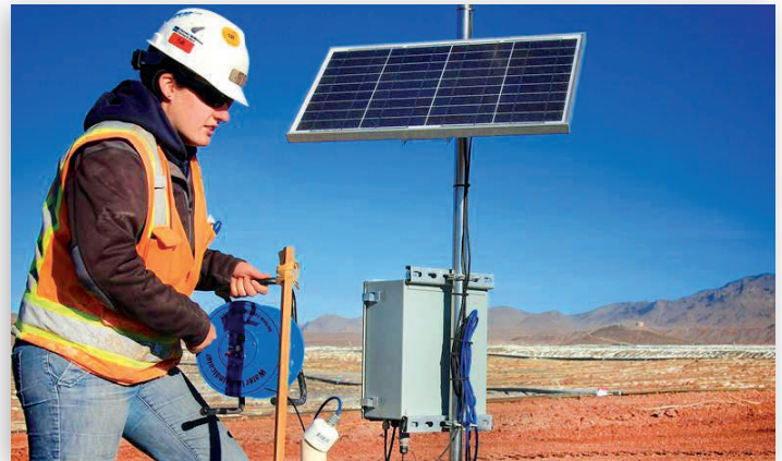
Karla Peabody, a metallurgist at the Safford operation in Arizona, maintains a piezometer on the Phase I leach pad. Piezometers provide real-time solution level data to metallurgists who monitor the structural integrity of leach pads to ensure the safe production of copper.
