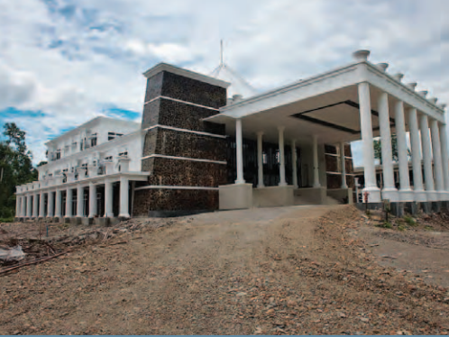
Tailings-aggregated concrete was used in the construction of the new Mimika Regency office near the PT Freeport Indonesia operations.
