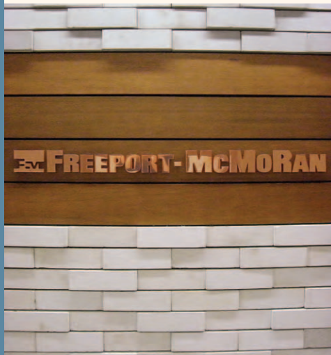
Bricks made primarily from tailings material decorate the lobby and elevator banks of Freeport-McMoRan’s new headquarters building in Phoenix, Arizona.
